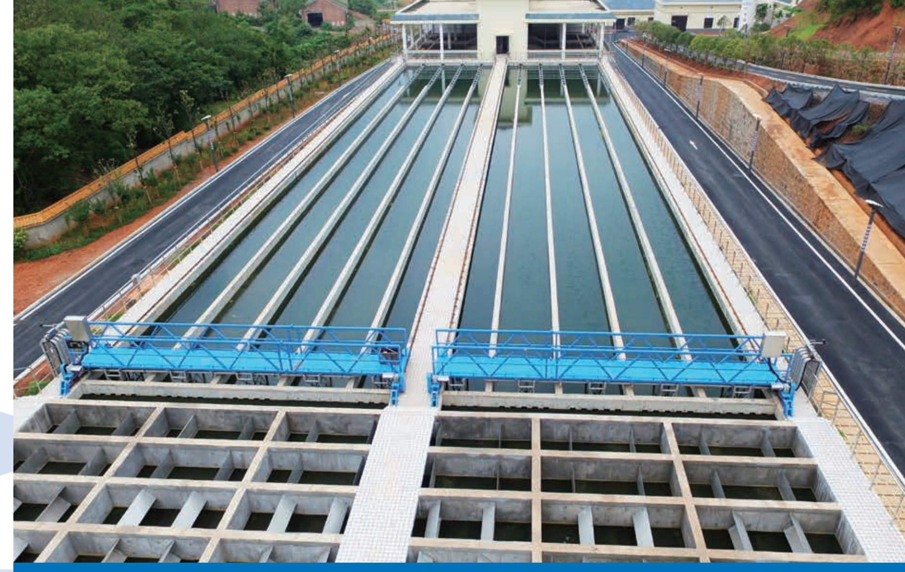
Drinking Water Plant
